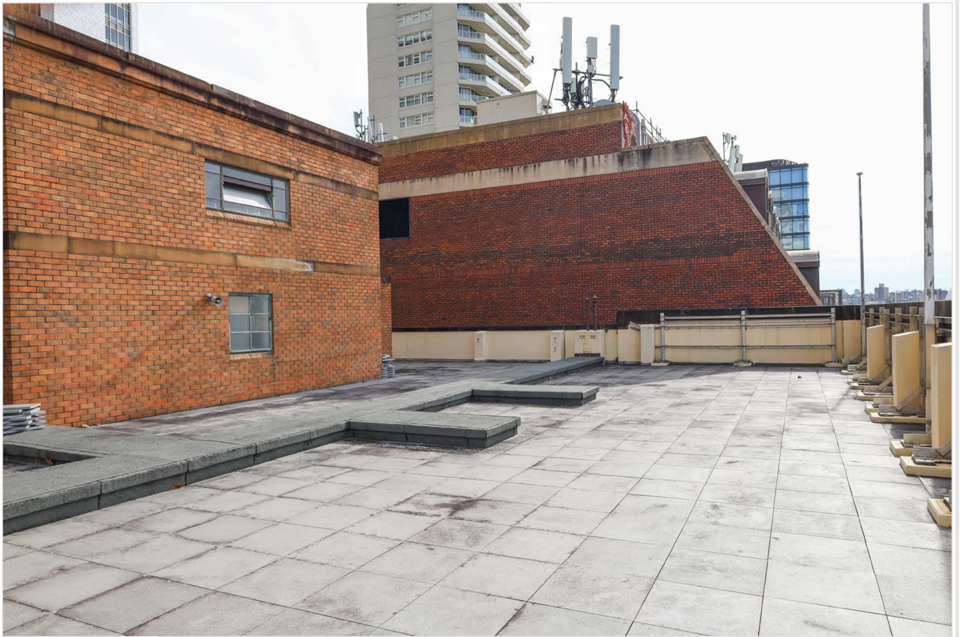
Existing site photo Intercontinental Hotel: - adjoining rooftop
